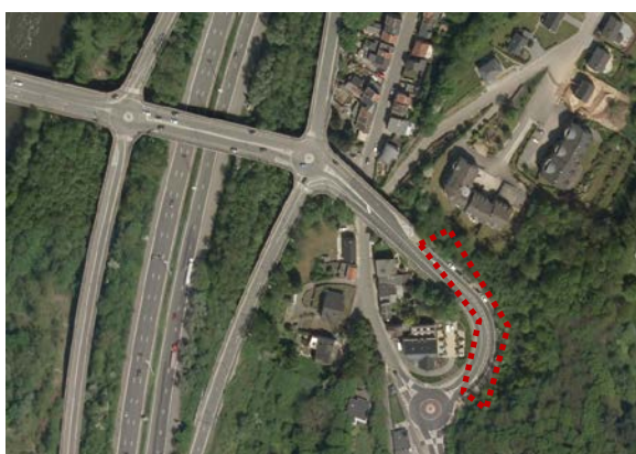
Photo 22. Parking de covoiturage N609
