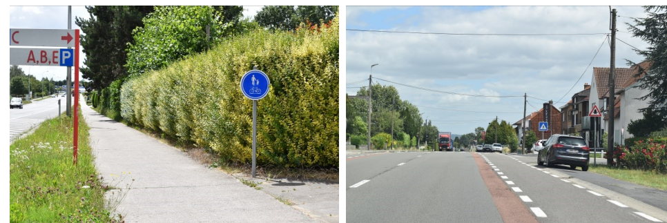
Photo 1: N513 / Photo 2: N512
