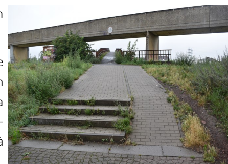
Figure 27: Passerelle rue Edmond Isaac
